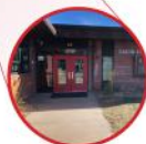
Eaton Elementary Decommission
